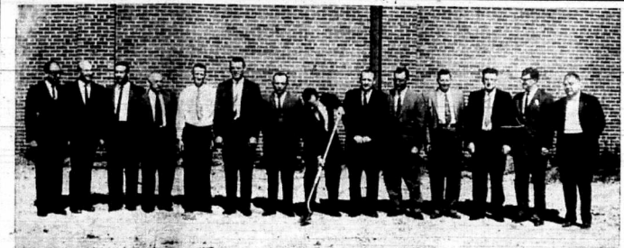
They turned the first spade of dirt for the new $600,000 Rowan County High School building on which work started this week: From left: William Whitaker, manager radio station WCCR; Rev. B. W. Moore, Orlin Caldwell, Herb Christian, Charlie Adkins; Clyde Litton; Judge Carl Jones; Bishop Supp; Clifford Casady; Sam Litton, Jr.; Fred Calvert; C. E. Lewis; Ray Allen; and Publisher W. E. Gruber. Reverends Allen and Moore were co-chairmen of the campaign in which voters added 50 cents on each $100 assessment to construct the building and other improvements to its school system, to be announced later. The Rowan County News editorially spoke for the bond issue during the past four years. Most of the people are members of the Fiscal Court or the Board of Education.
