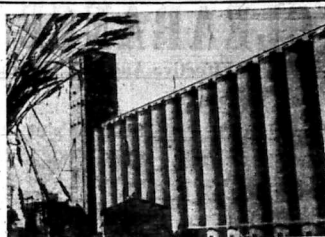
FARM AND FACTORY... The heads of wheat in the foreground will soon be reaped, then stored in huge grain storage elevators like these in Louisiana, Mo.
