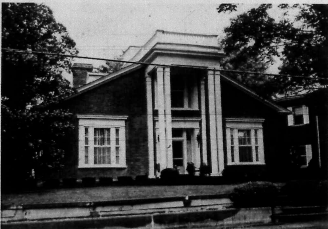
The historical home of Mrs. Henry R. Dicken is located on the highest point in Owingsville. Construction of the house was begun in 1839 and it was here that the Elder John Smith established Owingsville's first Christian
