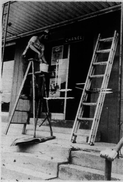
New Paint Job
