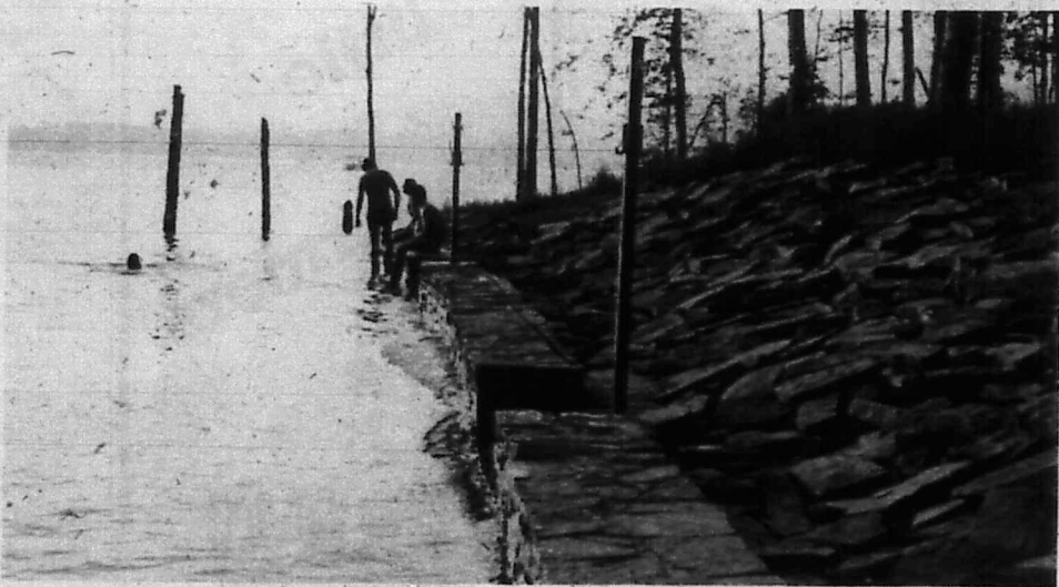
A spring flood turned this fishing point into a swimmers' dock. Fishing points with attractants in the water are
