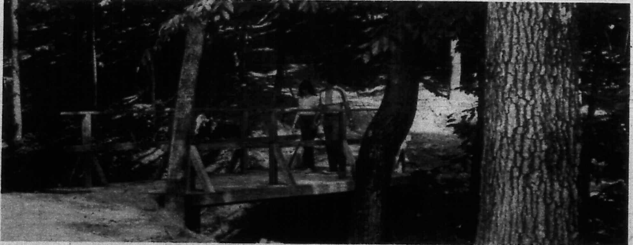
Danny Wise of Lewisburg and Peggy Lewis of Maysville stroll across the newly built bridge at Scott Creek Marina. The bridge leads to a graveled trail and a paved one being constructed for the handicapped. (Staff photo by Kathy Partin)
