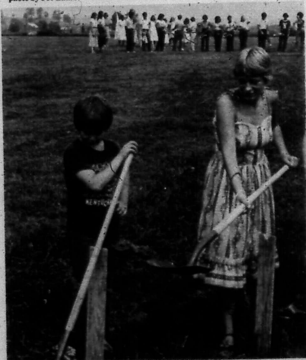
Vonda Ramey, sophomore class president at Rowan County High School, throws a spade full of dirt at the recent senior high school groundbreaking ceremony. Vonda's class is expected to be the first to graduate from the new building on the Old Flemingsburg Road. Bruce Hubbard, fourth grader at Farmers, represented all elementary students in the county. He didn't know he was going to be in the ceremony until a school official picked him up at school that day. (Staff photo by Kathy Partin)
