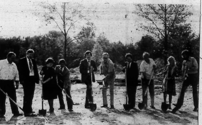
On hand Thursday afternoon to officially get a new apartment project underway were, left to right, Philip Lewis, president of Clearfield Manor Associates, LTD; Terry Simmons and Fay Hatcher, from the architectural firm that designed the project; Paul Blair, attorney for the developers; Charles Blankenship, Gordon Fogle and Tom Fern of Farmers Home Administration; Clayton Perkins, one of the developers; Debra Huft, from Farmers Home, and Morehead City Administrator Don Evans.
