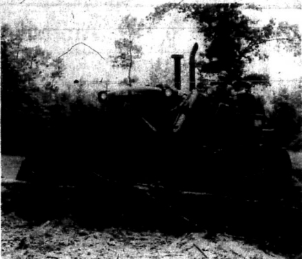
CLEAR ROAD — Spec. 4 Tony Jones of Morehead, a member of Company B, 201st Engineer Battalion, Kentucky Army National Guard, operates a bulldozer on a road clearing project at Camp Shelby, Miss. Company B, based in Olive Hill, is among 60 units in annual field training at this South Mississippi post. More than 2,500 Kentuckians are training at Camp Shelby this month.
