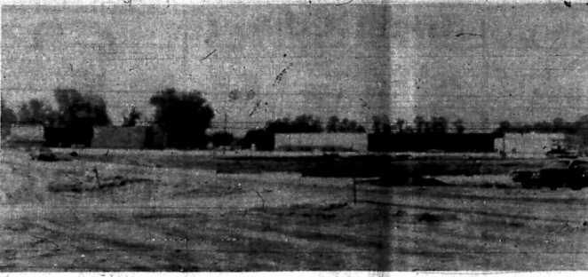
THE NEW HECK'S BUILDING is on the right and the new Thompson's IGA is on the left on North Mayville Road. Mr. Sterling, at the I-64 interchange. "We expect to be finished sometime during early September," Bill Leake, Construction Manager for the developer, E.M. Singer said. Leake said since the parking lot will have entrances on both U.S. 60 and the new bypass, the stores can open whether or not the bypass is finished.
