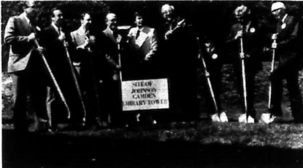
LOOK FOR THE YOUNGEST PERSON in this picture. This was the scene Tuesday when ground was broken for the Johnson Camden Library Tower expansion on the MSU campus which will cost $2.65 million. Johnson Camden Library was erected in 1930 and named for the late U.S. Senator Johnson Camden, a close associate of the late Senator Allie W. Young. Johnson Camden was married twice, and research started four months ago to find his nearest living relative to participate in this ceremony. The nearest relative is 10-year-old Johnson Camden Clay, a grand stepson of Paris, Ky. The boy dug his spade into the ground with determination which drew applause from the on-looker crowd. From left - Architect Louie Hugg; Dr. Jack Ellis, director of MSU libraries; Richard Lewis, Administrative Assistant to Gov. Julian Carroll; Dr. A.D. Albright, Chairman of Kentucky Council on Public Higher Education; Russell McClure, Kentucky Commissioner of Finance and formerly of Morehead; Dr. Adron Doran, the star of the show, Johnson Camden Clay; William Scent who was Finance Commissioner when funds were approved for the library project; Dr. William H. Cartmell, Chairman of the Board of Regents. This is the second time that Johnson Camden Library has been expanded since 1930.
