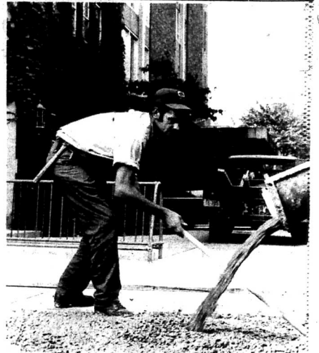
SMOOTHING THE WAY... Morehead State University workman Jimmy Dehart of Rt. 2, Morehead, spreads concrete inside a sidewalk form as MSU's maintenance staff prepares for the opening of school on Monday. Registration runs through Wednesday and classes start Thursday.
