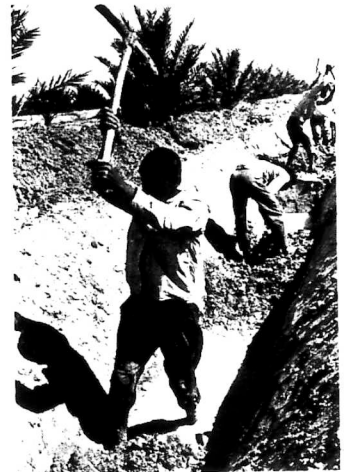
Digging a drainage ditch for irrigation project in southern Tunisia. (World Bank photo)
