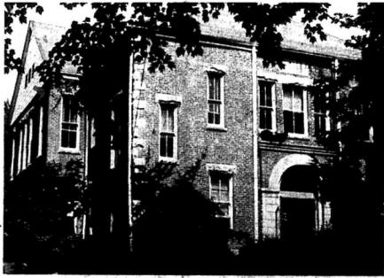
IF THESE WALLS COULD TALK . . . This is the 85-year old courthouse at Morehead. The condemned jail, not shown in picture, is at right. The old courthouse will be vacated by February and offices moved to a site on the I-64 connector, purchased with building Tuesday by Fiscal Court for $700,000.
