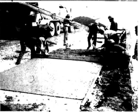
BUILD SIDEWALKS. Corpsemen from the Pine Knot Civilian Conservation Center construct sidewalks at the swimming beach at the Twin Knobs Recreation site on Cave Run Lake.
