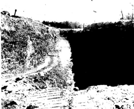
BURIAL SITE. The newest burial trench at Maxey Flats in Fleming County where Nuclear Engineering Company disposes of radioactive waste materials is about 50 feet wide, 30 feet deep and 650 feet long. During the past 12 years, an estimated 18 acres have been used at the Maxey Flats site for burial of nuclear waste.
