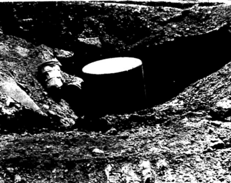
NUCLEAR DISPOSAL SITE. Materials contaminated with radioactive elements are shipped to the Nuclear Engineering site at Maxey Flats in Fleming County where they are buried in trenches like that pictured. (Another picture on Page 2.)
