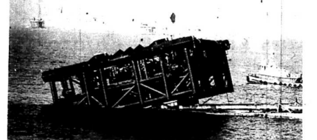
Exxon USA's prototype Submerged Production System is launched from a barge 27 miles southeast of Grand Isle, Louisiana. The unit, designed to produce oil and gas with remotely-controlled, ocean floor equipment, has been lowered to the sea floor in 170 feet of water for an extensive testing period. The test project, representing more than 300 man years of research and development and an investment of $30 million, is presently designed to operate in water depths to 2,000 feet. Objective of the FPS program is to develop a petroleum production system for water depths beyond the economic and technical limits of platforms.
