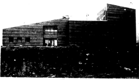
DEDICATION SET - The 12,000 square foot brick veneer structure that will house the permanent archives and activities of the Kentucky Democratic Party stands near completion on I-64 at the U.S. 60 interchange, just outside Frankfort. Official dedication ceremonies will be held Feb. 22 at 2:30 p.m. CDT.
