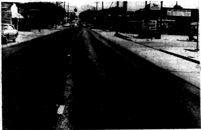
RESURFACING MAIN STREET . . . Morehead's Main Street looks like this today as the center lanes have received a prime coat of resurfacing. Scheduled within the next two weeks is complete resurfacing the street all through the city. This cannot be done until culverts and manholes are elevated to meet the new (higher) street surface. The middle prime coat, as pictured, is necessary for good drainage and compactness.
