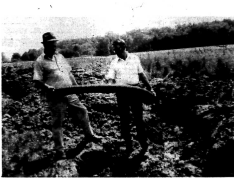
"It sure doesn't look like tile," L.G. Bishop, left appears to be telling D.L. McDavid, Conservation Technician with the U.S. Soil Conservation Service. Actually, Bishop and McDavid are examining a section of corrugated polyethylene drainage tubing. In the background are trenches in which 3100 feet of this new drainage product was installed to lower the water level and increase productivity of this field on Mr. Bishop's Triplett Creek Farm.
