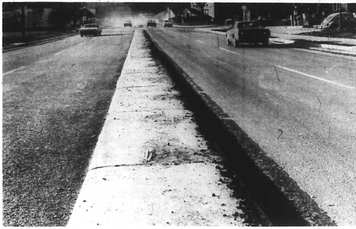
PAVED BEFORE DEADLINE... The Bizzeck Construction Company, prime contractor for the 2.8 mile I-64 connector at Morehead, raced the clock last week to ready the stretch for winter travel. Deadline for laying blacktop in Kentucky is November 15. Now, all lanes are open to travel. However, what you see is not the completed job. Come spring this
