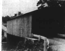
LEE'S CREEK BRIDGE ... at Dover in Nelson County
