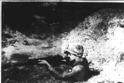
PORTSMOUTH ROOF — Behind this soldier is a foxhole cover supporting 36 inches of top soil. Pleasantly being tested by the U.S. Army Infantry Board, Fort Benning, Ga., the cover measures 80 by 84 inches and is made of close-woven daron. It has two eight inch sleeves, one at each end, which can be filled with soil and buried to serve as anchors. The cover weighs less than two pounds and can be folded into a seven by seven and a half inch portable packet.
