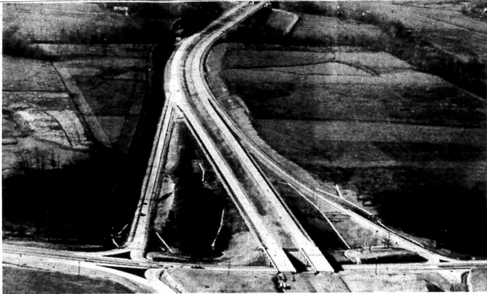
DEDICATION TUESDAY... This is an aerial view of the I-64 interchange at Morehead which will be dedicated and officially opened to traffic next Tuesday (Nov. 17) morning. A portion of I-64 in Carter County will have its ribbon cutting Tuesday afternoon.
