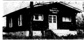
NO SMOKING? . . . People seeking the Chamber of Commerce offices at Middletown, Ky. are directed to the "cool house" near the highway. Middletown officials used coal as building material to promote the image of coal in the area.
