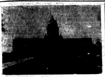
Front view of the Kentucky State Capitol at Frankfort. Necessary repairs amounting to $68,000 are being made to the dome.
