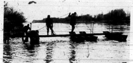
BRIDGE ACROSS THE DANUBE —U.S. Army soldiers erect an aluminum floating footbridge over the Danube River near Grossmehring, Germany, in assault exercise conducted by Company D of the 78th Engineer Battalion. Despite the river's seven-foot-per-second current, the engineers laid the footbridge for the assault exercise with no trouble.
