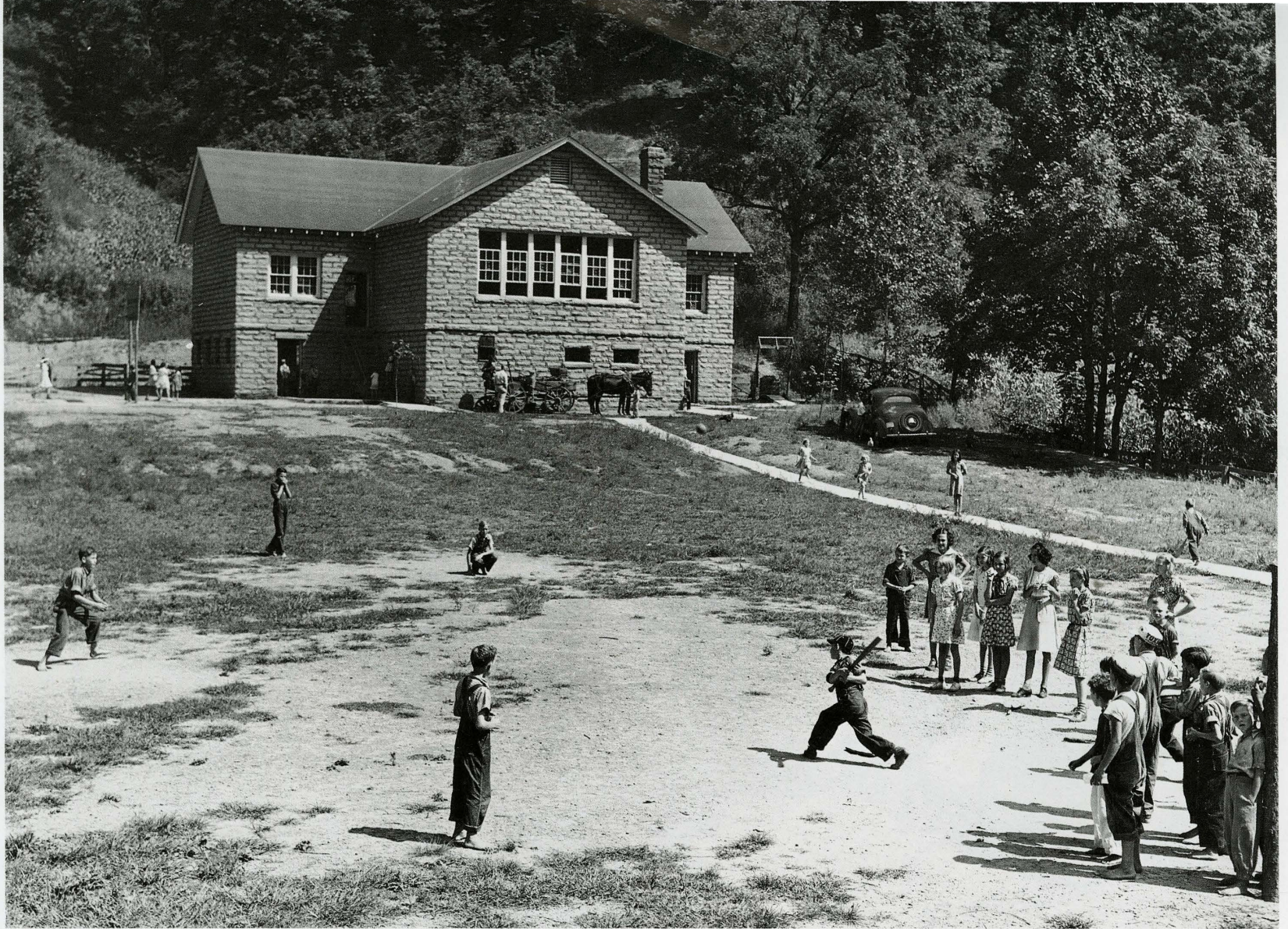
Softball near Big Rock school, one of the new consolidated schools being constructed with federal assistance. Superintendent Marie Turner wanted them built of stone because so many wooden schools had burned. Breathitt County, September 1940. MARION POST WOLCOTT.
