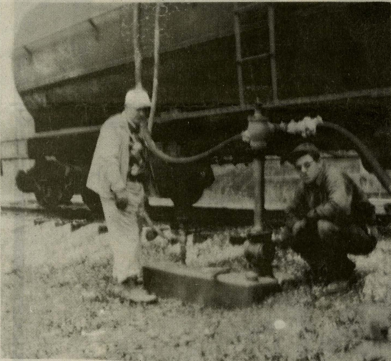
Casual Linville (left) and Jim Williams pump "LP" Butane gas from railroad car to Williams-Nickell tanks.
