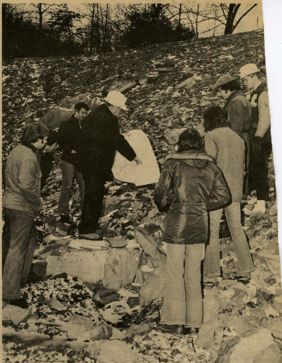
IN THE FIELD . . . Orris Watson, associate professor of mining technology at Morehead State University, explains the construction and purpose of a silt dam to students at a strip mine in Carter County. MSU has two associate degree programs in the mining industry, mining technology, and reclamation technology. Both involve extensive field studies.
