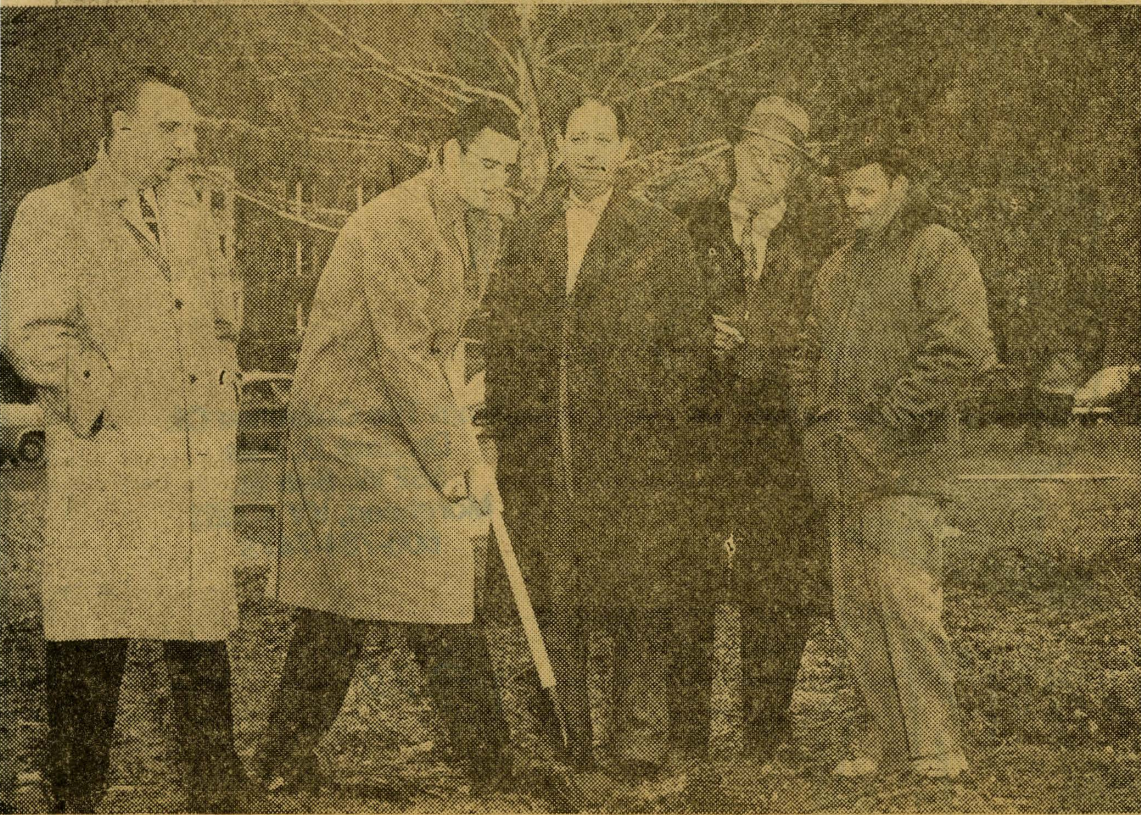
STUDENT COUNCIL PRESIDENT Steve Hamilton was given the honor of turning the first spade of dirt for the new $725,000 Doran Student House at Morehead College. Looking on are Dean Roger Wilson, President Adron Doran, Supt. of Buildings and Grounds W. H. Rice and the contractor.
