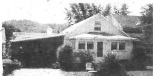
6 ROOM FRAME DWELLING fronting on Fleming Avenue and Flemingsburg Road. Lot runs from street to street. Utility room, boxed off attic upstairs for storage and sleeping. Large patio-carport on Fleming Avenue entrance. Tiled floors throughout. Fireplace in living family room off the kitchen. Good size lot 52 feet on both sides and approximately 150 feet through. Priced at only $16,000.00.
