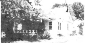
3 BEDROOM STONE VENEER DWELLING with full basement, 1 car garage in basement, beautiful built-in kitchen cabinets and dining area. Living room and bath. Central heat in basement. Large lot in Alfrey Heights Subdivision in city of Morehead. Priced for quick sale at $15,000.00.
