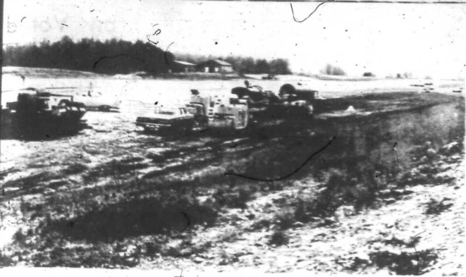
SMOOTH STRIP — The landing strip of the Morehead-Rowan County Airport at Farmers this week was getting final touches of blacktopping with only a parking apron remaining to be surfaced. The runway is now open to aircraft. Blacktopped at a cost of $94,000, the 2,900-foot strip is now ready to be lighted and with completion of this phase the airport will be the finest and most modern in the area. Lewis and Clark is the contractor on the job.
