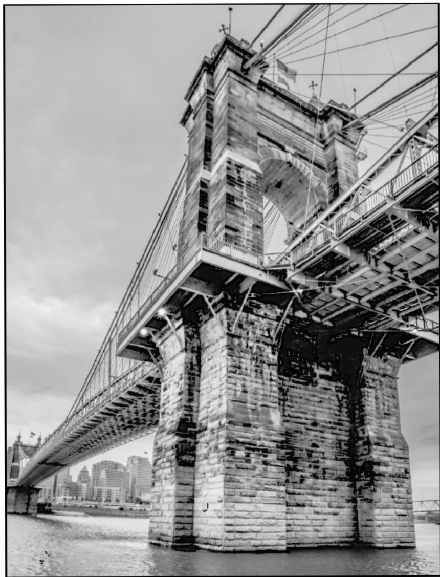
Christopher Burton Bridge Black and White Photograph
