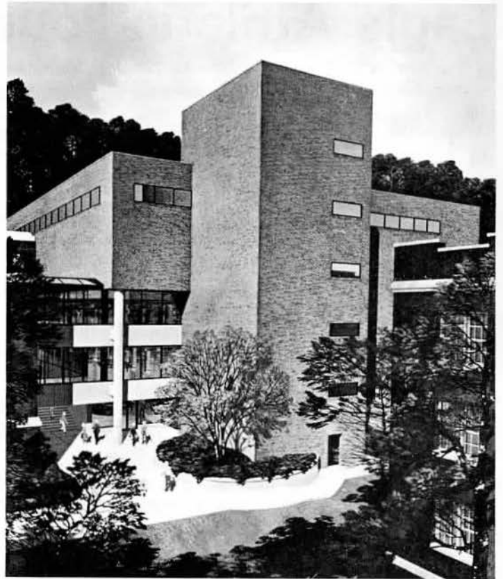
TOWER FINISHED—"To Honor a Great Kentuckian" will be the theme of the dedication of MSU's Julian M. Carroll Library Tower on Saturday, Oct. 21, at 11 a.m. The $2.5 million facility adds 40,000 square feet of floor space to MSU's Johnson Camden Library. The dedication ceremony is open to the public.
