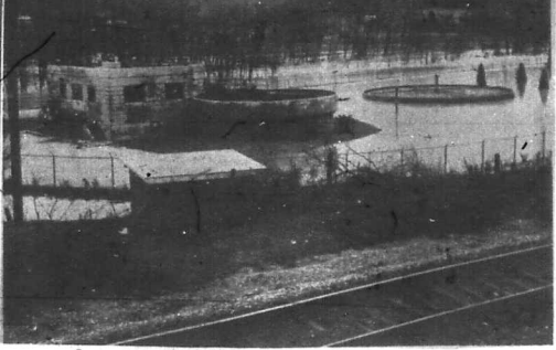
Overflows Sewage Plant SURFACE WATER - The runoff from Sunday's thunderous downpour sent Triplet Creek, and its tributaries, to their banks in much of this section. Water from the main stream itself leaped out of the normal confluence of the creek and spread rapidly to lower sections. The Morehead Utility Plant Board's sewage disposal plant was almost surrounded late Sunday when Triplet overflowed near Clearfield. Although the rainfall was the heaviest for such a short period since 1939, damage was slight.
