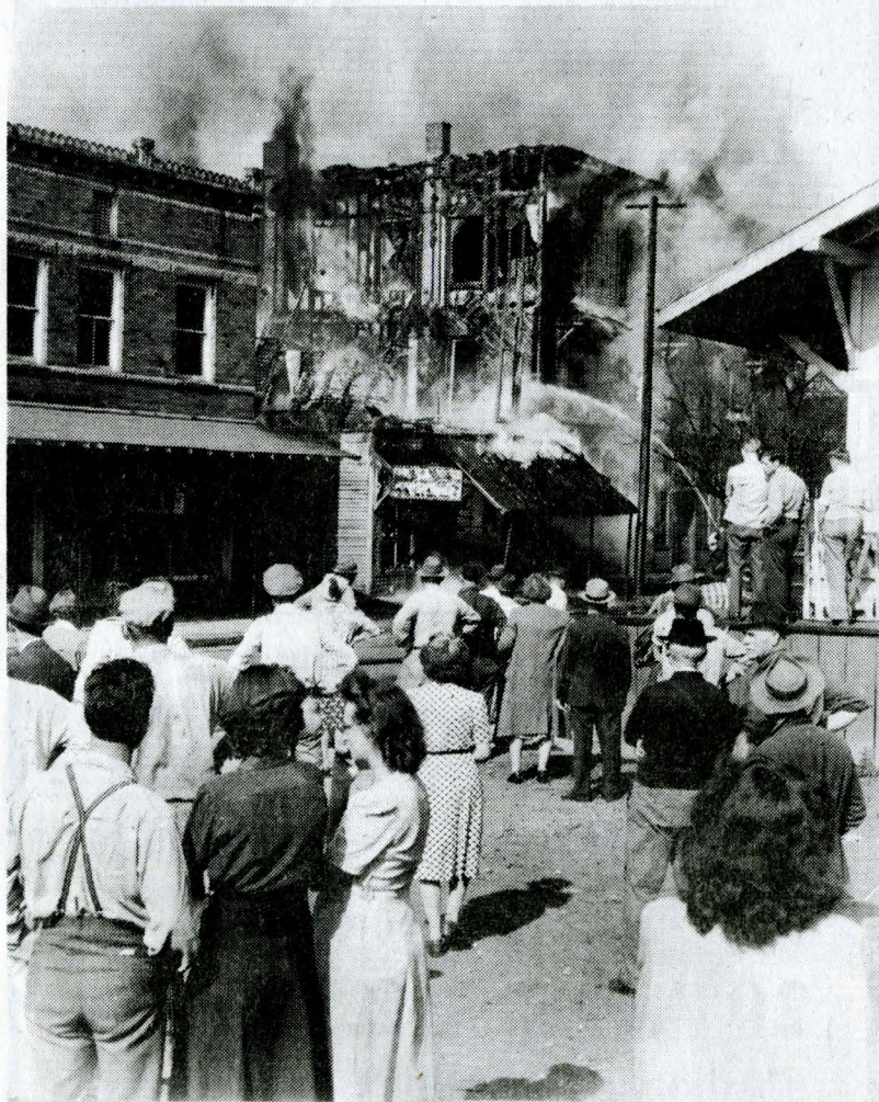
In November 1946, Morehead firefighters battle a fire on First Street. The three-story wooden People's Hotel, owned by Ezra Proctor, and the one-story store building, owned by Sam Allen, were completely destroyed. However, the Big Store, left, and the Freight Station, right, were saved. (Photo courtesy of Roger and Bernice Barbour).
