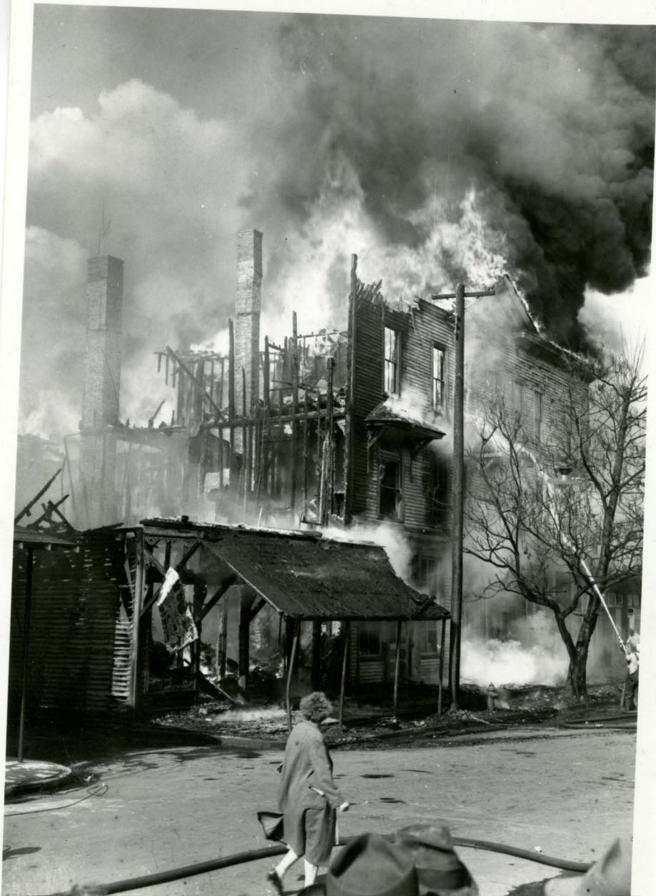
LANDMARK GOES DOWN. The Peoples Hotel on First Street was once a center of activity and the walls could tell many tales about early life in Morehead. The hotel was destroyed in this fire November, 1946. Sam Allens Store was also destroyed. Photo: Art Stewart
