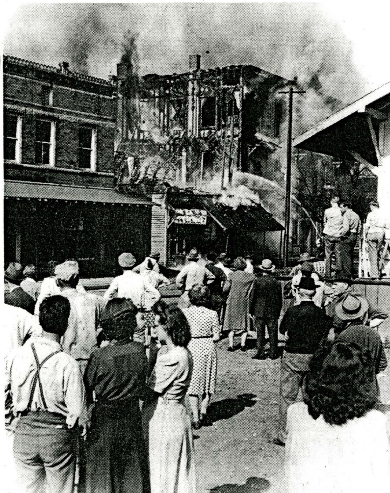
In November 1946, Morehead firefighters battle a fire on First Street. The three-story wooden People's Hotel, owned by Ezra Proctor, and the one-story store building, owned by Sam Allen, were completely destroyed. However, the Big Store, left, and the Freight Station, right, were saved. (Photo courtesy of Roger and Bernice Barbour).
