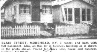
BLAIR STREET, MOREHEAD, KY. 3 rooms and bath with full basement. Also, on this lot is business building as is shown in the photo above. Priced for quick sale, house and business building $10,000.00.
