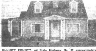
ELLIOTT COUNTY , on State Highway No. 32 approximately 3 1/2 miles from Sandy Hook and 24 miles from Morehead. 1 1/2 story frame, Cape Cod Dwelling, 4 bedrooms, living room, kitchen and family or dining room. Good dry basement. Storm windows, drapes, blinds, carpets in two rooms, almost new stove in kitchen. Built-in cabinets in kitchen. An attractive country home on good lot fronting on blocktop Road 100 feet and extending back a distance of 150 feet. Priced at $14,000.00.
