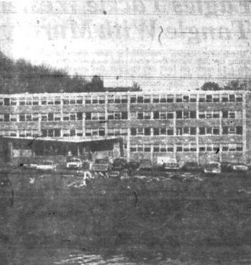
REGENTS HALL - Morehead State College's new dormitory, Regents Hall, opened last week. The $725,000, ultra-modern structure is completely air-conditioned and will serve as an honors dormitory. It will house over 200 male students.
