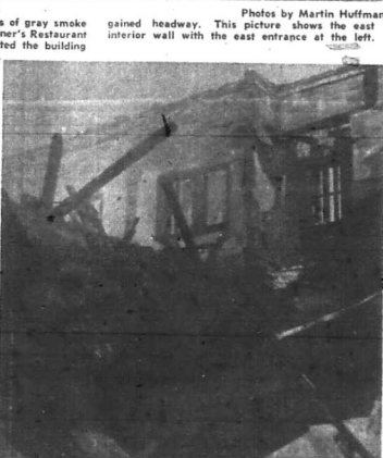
THE AFTERMATH — This was the scene Friday morning as the ruins of what had been one of Kentucky's most unique restaurants, continued to smolder. Only exterior walls, constructed of masonry, remained standing. Fire department personnel spent another two and one-half hours at the scene Friday after smoldering ruins burst into flames once more.
