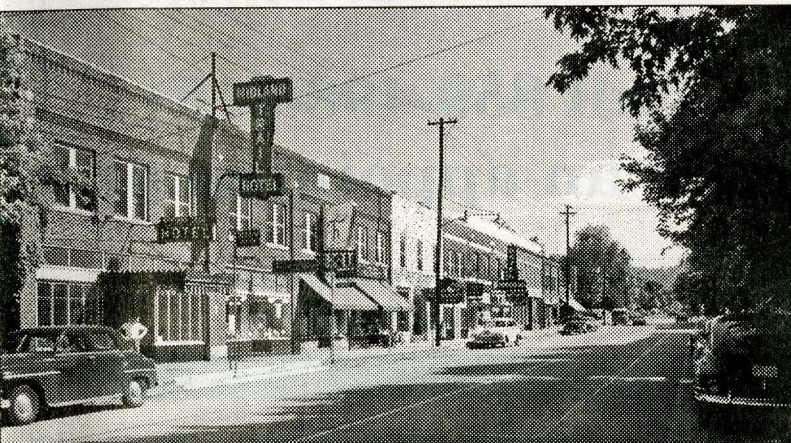
Morehead's New Mains Street had shown great progress in 1945.
