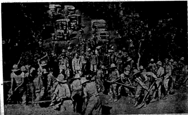
Italian engineers are constructing roads in Ethiopia for the use of the Italian forces. Recent rains have destroyed many of the roads that were built by the Italians, according to reports.
