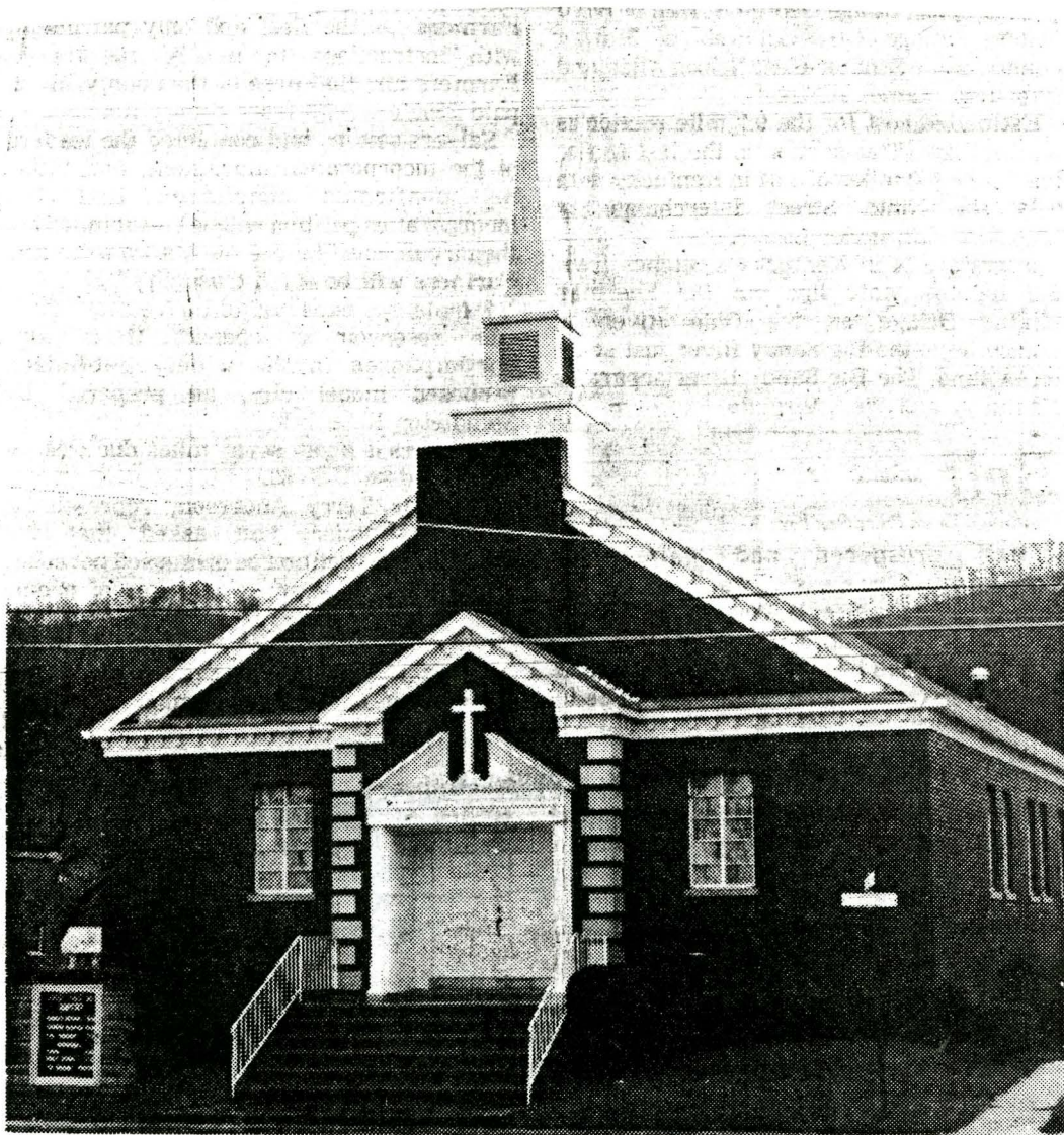
A STEEPLE WITH A BELL . . . The steeple on the First Freewill Baptist Church on Morehead's west Main Street has been completed and a 113 year old bell, used in Morehead's first city hall, installed. The carefully preserved bell, contributed by 98 year old Norman Wells, sounded Sunday for the first time in 53 years.
