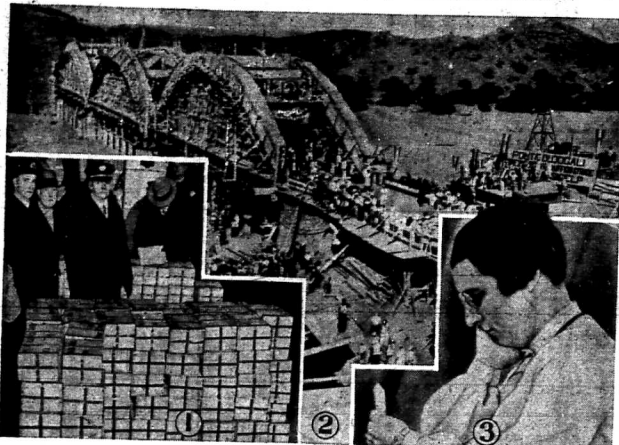
1—Millions of dollars in gold being unloaded from the liners Majestic and Alaunia at New York. 2—Massive bridge across the Enteclo river in Ethiopia being constructed by the Italian army. 3—Mrs. Elliot Evans of Chicago, woman member of the team that was the national mixed pair championship in the American Bridge League tournament in Chicago.
