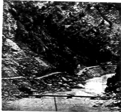
Looking into the canyon of the North Platte river in Wyoming, where the Seminole storage dam, the main link in the Casper-Alvora reclamation project will be erected. Planned to stand 200 feet tall, the dam will be the "border of the Northwest." The footbridge in the foreground is located at the approximate upstream toe of the dam.
