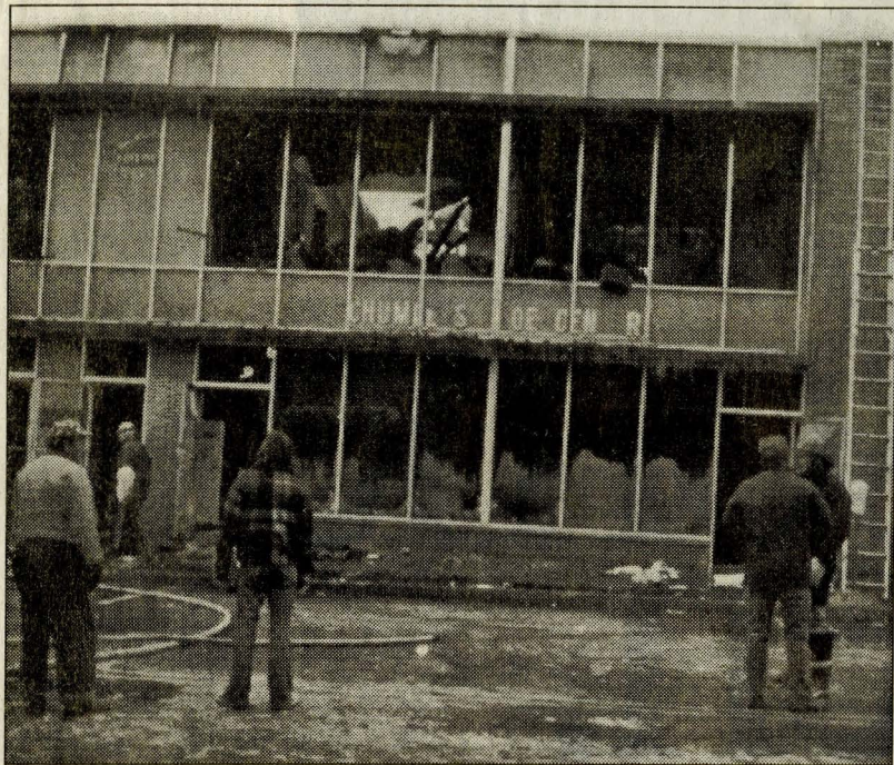
Morehead firemen survey devastation caused by fire that destroyed Chumley's Shoe Center and the Lewis Building December 1975.
