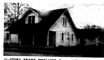
1 1/2-STORY FRAME DWELLING , 7 rooms, 1 1/2 baths, 4 bedrooms, gas radiators, all utilities. Corner Branham and Railroad Street. Can assume a V.A. guaranteed loan of approximately $4,000.00 payable $66.00 per month including taxes and insurance.
