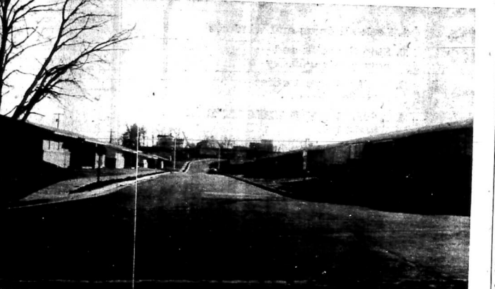
NEARLY SAME — This is the 84th Terrace Housing project in Mt. Sterling, which Morehead's low-rent housing project will closely resemble when it is completed next month. The contract for the local job was let last week and work is to start prior to June 17. Brick and frame construction will be used. Rents will range from $36-53 monthly.
