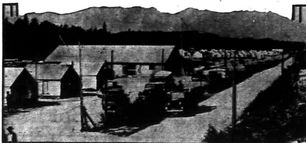
The town of Palmer, being built in Matanuska valley, Alaska, by colonists from the Middle West, is pictured here on a busy day. In the foreground are the administrative headquarters of the Alaska Rural Rehabilitation corporation. The long building is the warehouse which also houses the telegraph and radio offices of the United States army signal corps. Tents of the colonists are to be seen in the background.
