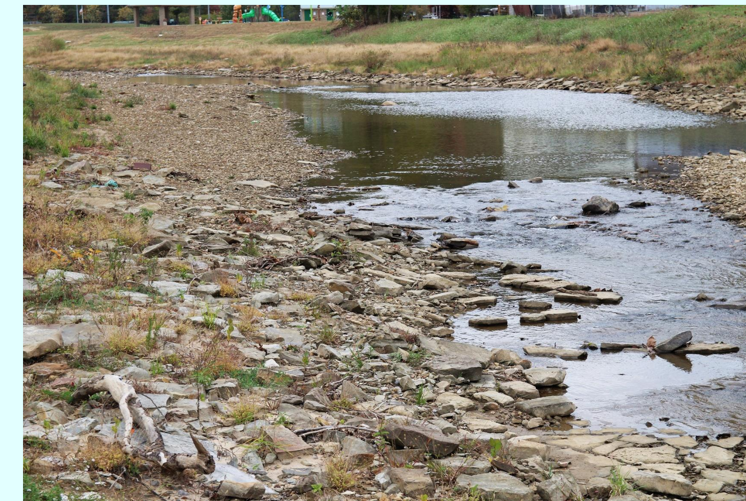
Figure 4. Upper Restored site after restorations (October 2019).
