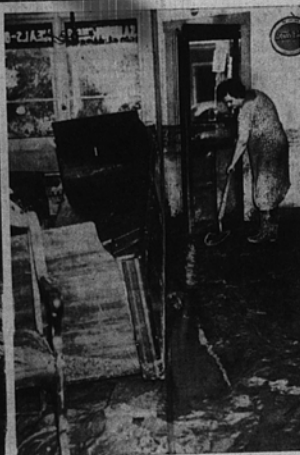
4 FLOOD MUD . . . Mrs. S. B. Mutters began shoveling the mud and debris out of her restaurant at Morehead as soon as the waters rolled away.
